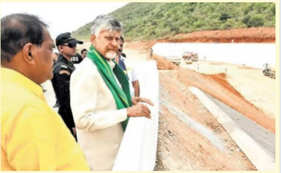
oversee the subsequent stages of water conveyance. On Monday, Chief Minister Chandra babu will officially release water from the Veligonda project and dedicate it to the public.
